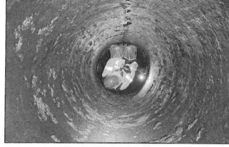
Removing bar screen for inspection
