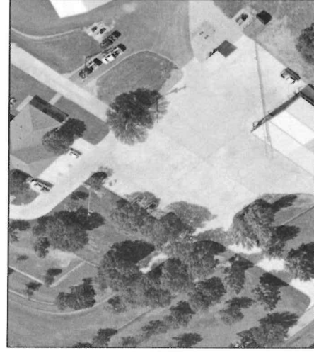
Office parking lot replacement
